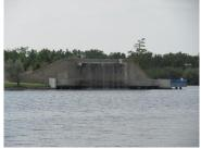
The waterfall trough is fastened to an existing cast in place concrete bridge abutment and a walkway passes underneath the waterfall. It consists of galvanized steel HSS 102X102 at 1350 on centre, wide flange beams,
