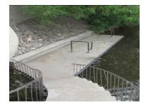
good condition. The slab on the mainland is cracked and the concrete bench on the slab is also cracked. The railing down to the dock is damaged and requires repair. Mooring posts on the mainland slab are loose and require tightening.
