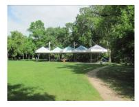
monitor. Four triangular steel columns hold up 12 fibreglass hexagon shaped canopies. Connections between the top of the columns and the roof panels are provided by steel rods with turnbuckles. The columns, rods and roof panels are all in good condition.
