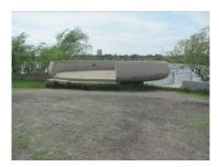
be removed at the entrance to minimize the step up to the overlook deck slab. The membrane protecting the concrete deck has worn and requires replacement. The concrete deck slab and perimeter wall is pocked and cracked. One of the stairs down to the lower concrete deck is severely damaged and requires replacement. The retaining walls adjacent to the structure exhibit vertical cracks at control joints and require sealant to prevent water migration.
