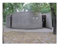
fluted face. The roof is also cast in place concrete. The three steel passage doors are in good condition. There are two 36" diameter skylights in the building and they are in fair condition. The BUR roofing is in poor condition and should be replaced along with the associated flashing and trim.
