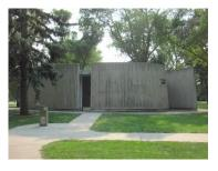
fluted face. The roof is also cast in place concrete. The paint on the three steel passage doors is worn and the wooden transoms are rotting and will soon require replacement. There are two 36" diameter skylights in the building and they are in fair condition. The BUR roofing is in poor condition and should be replaced along with the associated flashing and trim.
