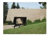
is precast concrete and is supported on the exterior walls and the interior concrete masonry block load bearing walls. The roof is partially buried and a membrane system is exposed and damaged in places. Exterior doors are painted steel and the finish has deteriorated.
