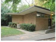
noted during the site visit and caulking at the masonry joints requires replacement. The roof is wood framed with built up roofing and is in fair condition however the plaster coating at the soffits needs repair. Wired glazing set in wood frames is cracked in at least three panels and the paint is worn. The three steel passage doors require repainting. There are two skylights in the building and they are in good condition.
